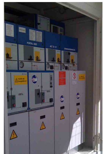
Gotthard Tunnel (Switzerland)
